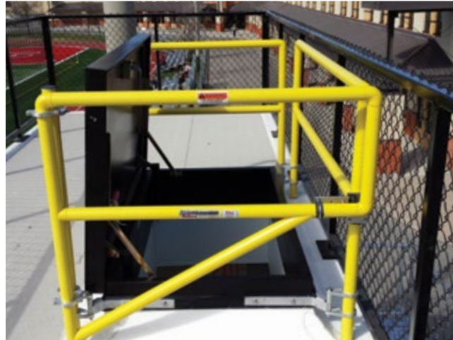
Roof Top Access Hatch with Interior Ships Ladder
